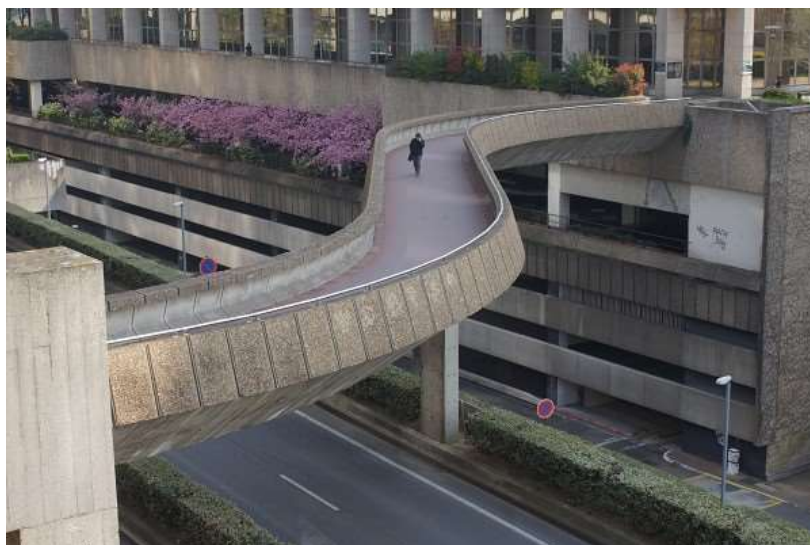
Passerelle Jean Moulin, Paris
